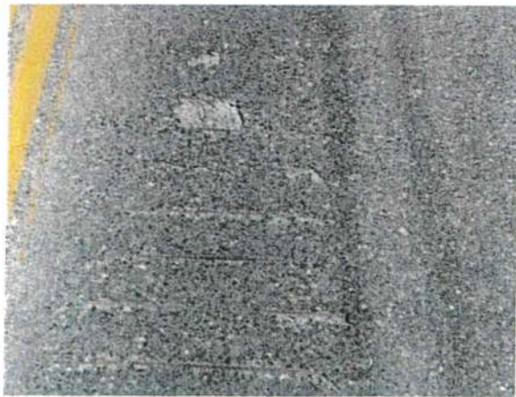
Galvin MP 1.55 Bridge #75
