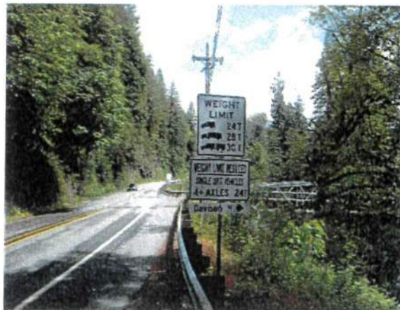
Davison Bridge #1 is posted with weight restrictions
