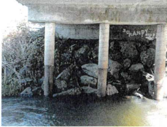
Senn MP 0.89 Bridge #77
