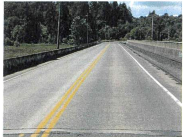
Galvin MP 1.23 Bridge #112
