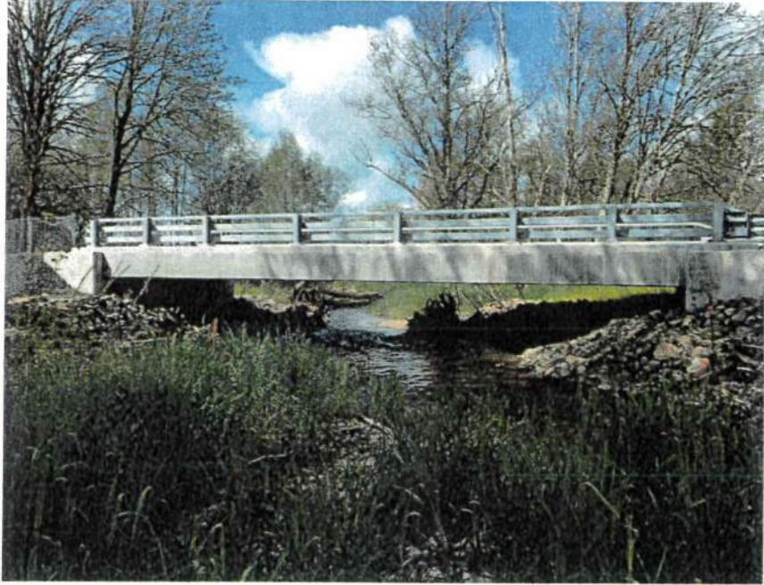
TOWNSEND MP 0.22, Bridge # 223 Post-Construction
