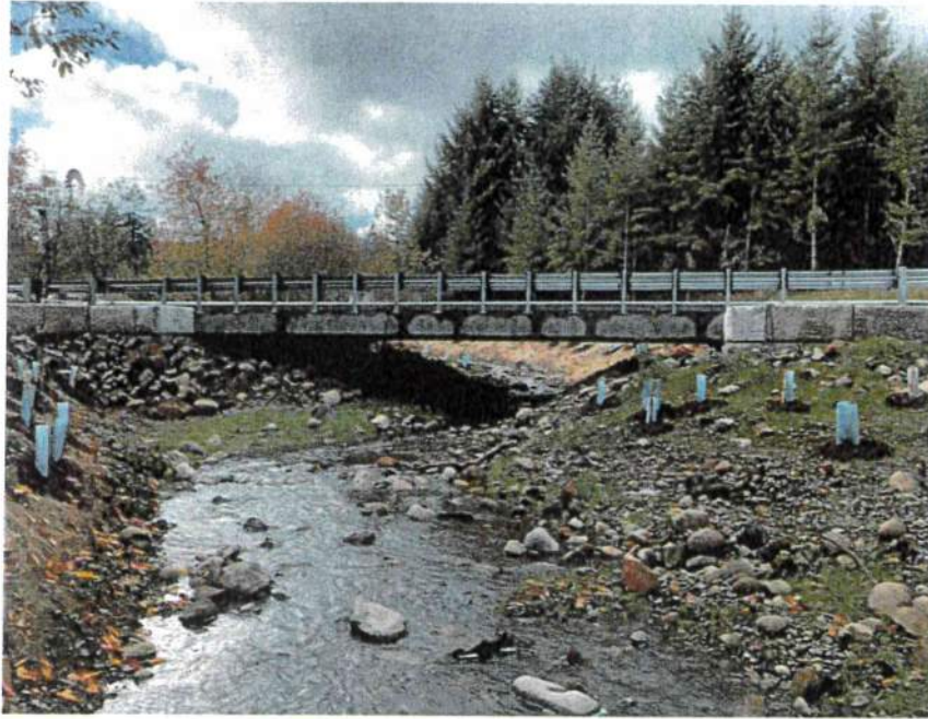
COUSINS MP 3.15, Bridge # 79 Post-Construction
