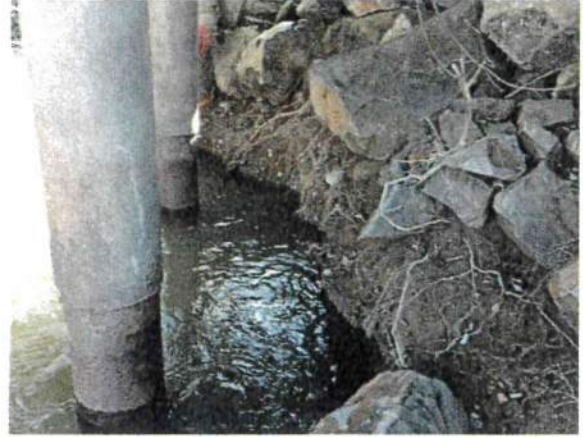
Senn MP 0.89 Bridge #77
