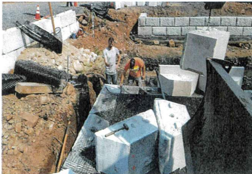
COUSINS MP 3.15, Bridge # 79 Mid-Construction
