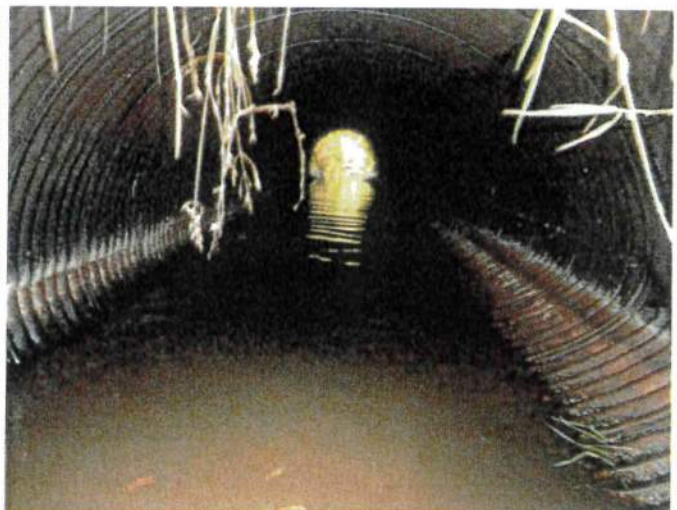
Centralia Alpha Road MP 15.79 inlet
