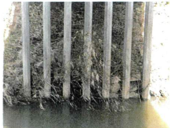
Wildwood MP 10.14 Bridge #3
