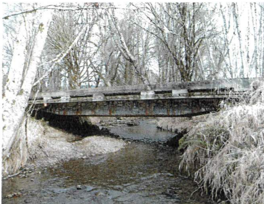
TOWNSEND MP 0.22, Bridge # 223 Pre-Construction
