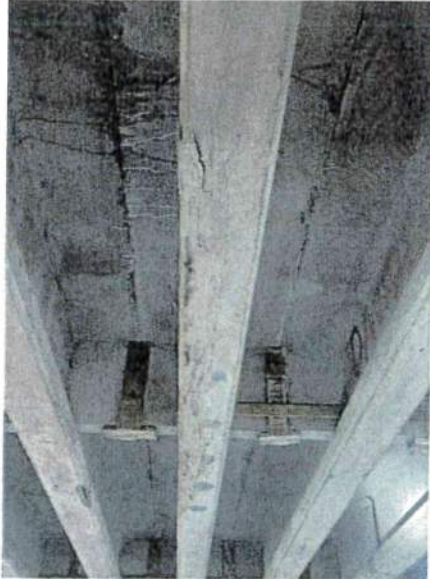
Hinning MP 0.23 Bridge #8
