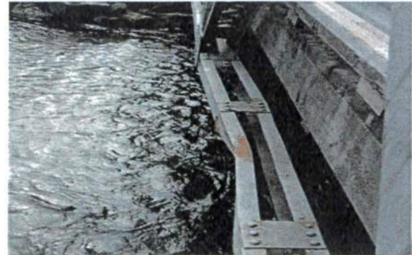
Davison MP 0.01 Bridge #1
