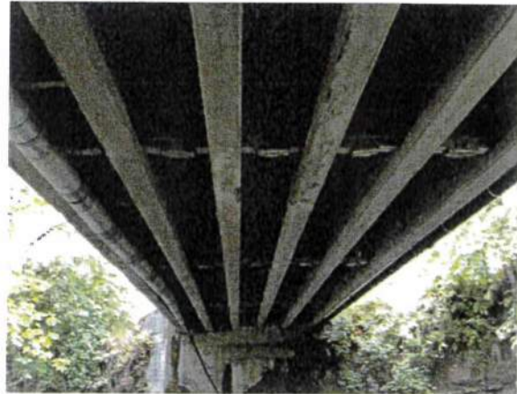
Hinning MP 0.23 Bridge #8
