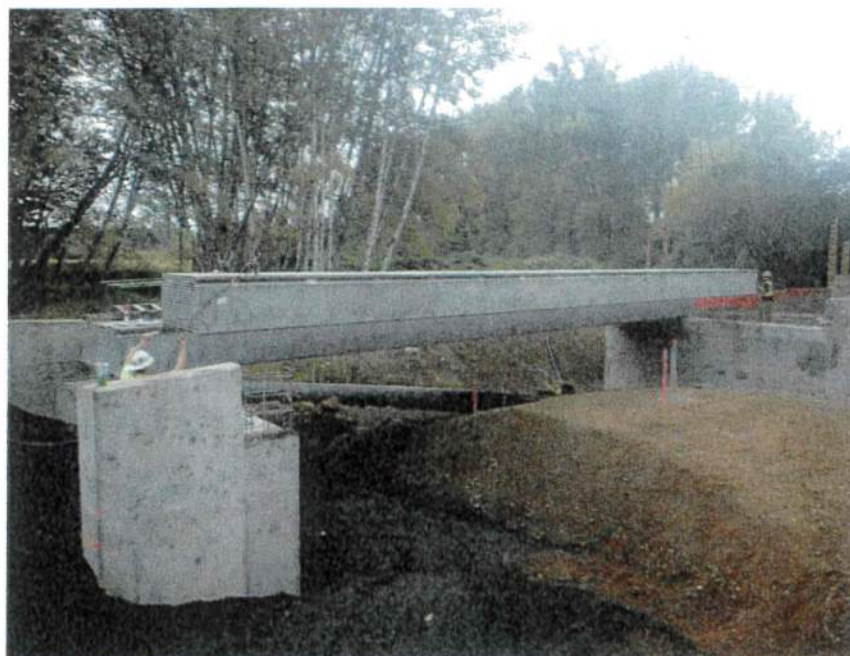
TOWNSEND MP 0.22, Bridge # 223 Mid-Construction
