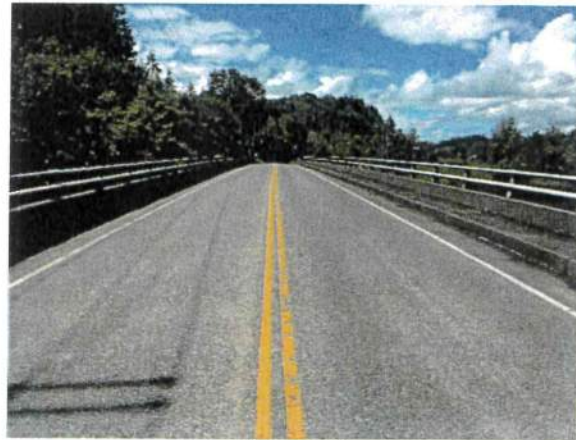
Galvin MP 1.55 Bridge #75
