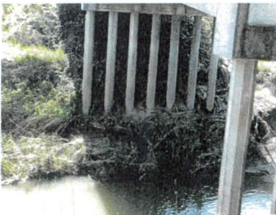
Wildwood MP 10.14 Bridge #3
