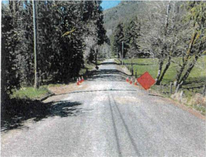
Crumb Road MP 0.17 roadway above culvert
