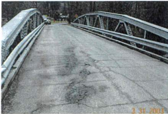
Davison MP 0.01 Bridge #1
