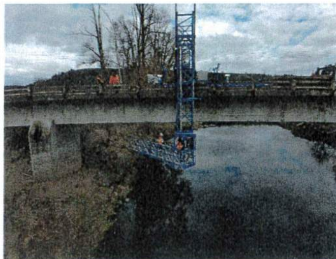
Ceres Hill MP 0.79, Bridge #102
