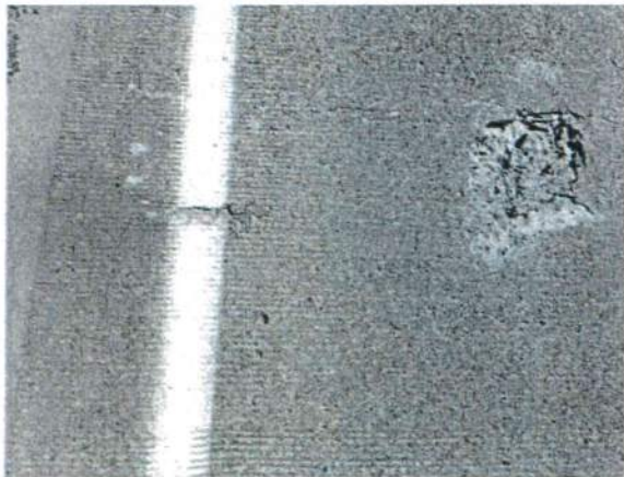
Galvin MP 1.23 Bridge #112
