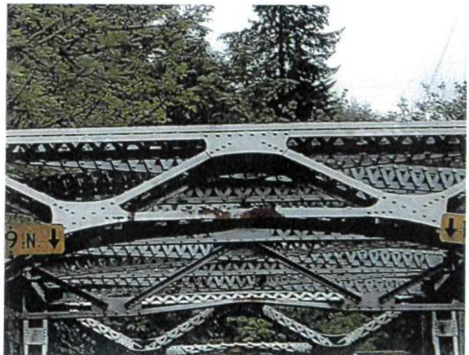
Ferrier Bridge #93 bent portal bracing
