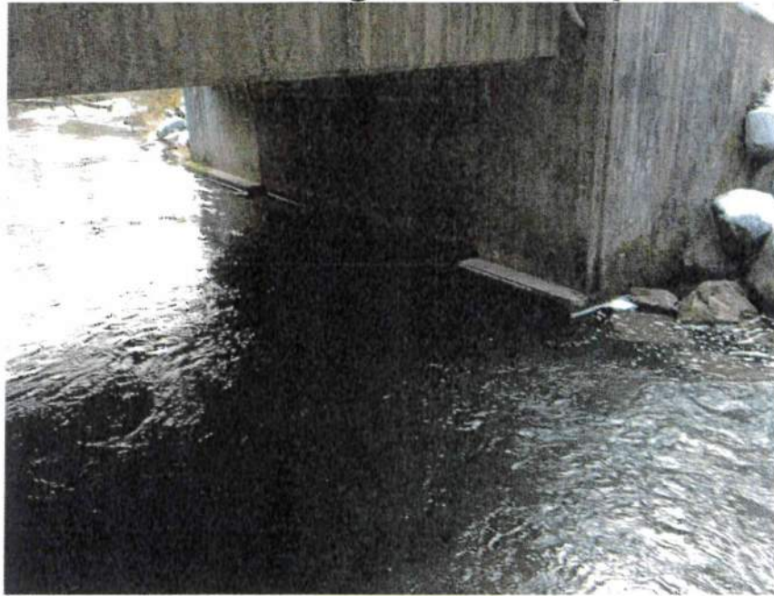
STOWELL MP 0.57, Bridge # 221 Pre-Construction
